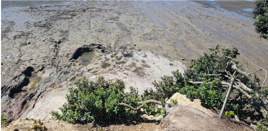
Figure 2. Point at the base of the cliff at 38 Rawene Ave
